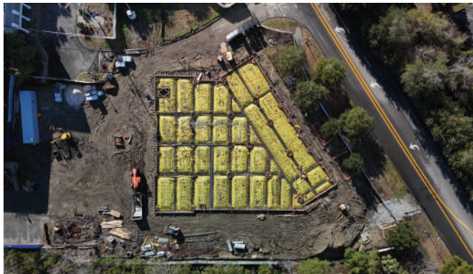
SETUP Evans Contracting Group gears up to pour a 650-cu-yd slab at Mediterranean Shipping Co. headquarters in Mount Pleasant, S.C.
